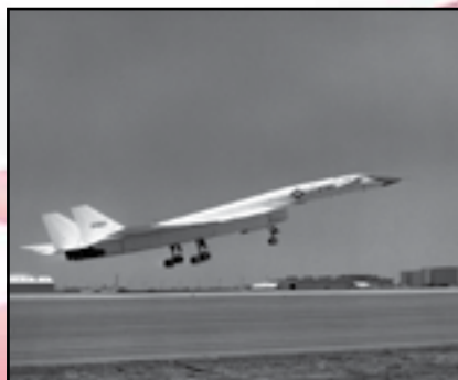
Oct. 12, 1964: The North American Valkyrie reached supersonic speed (Mach 1.11 at 35,080 feet) for the first time during its third flight. North American test pilot Al White reported a smooth transition from subsonic to supersonic flight.
